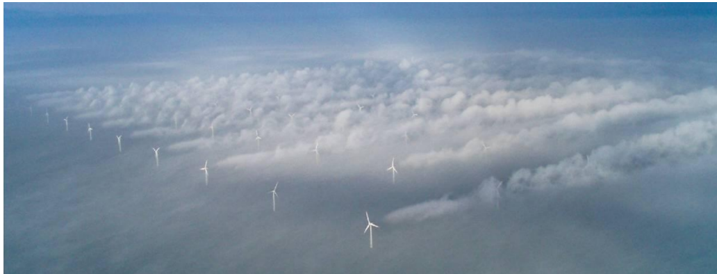
Figure 4. Photograph of the Horns Rev 1 wind farm (12/02/2008 around 10:10 UTC) from southeast. Courtesy Vattenfall. Photographer: Christian Steiness
