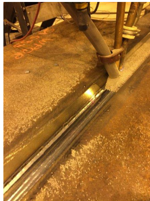
Figure 1: SAW process (121) being done on coupon in SA-533 type E material
